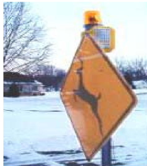
Figure 2. Enhanced deer crossing warning sign.
