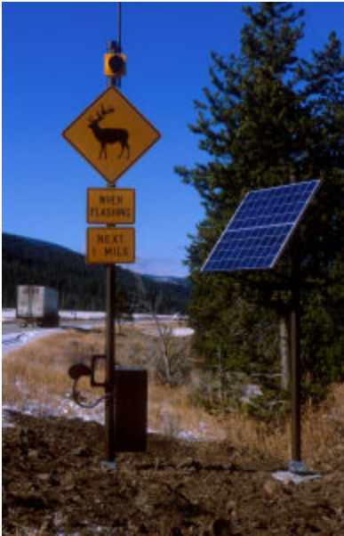
FIGURE 6 Dynamic elk sign and sensor system example ( Photo courtesy of the Western Transportation Institute ).
