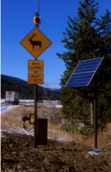
FIGURE 6 Dynamic elk sign and sensor system example ( Photo courtesy of the Western Transportation Institute ).
